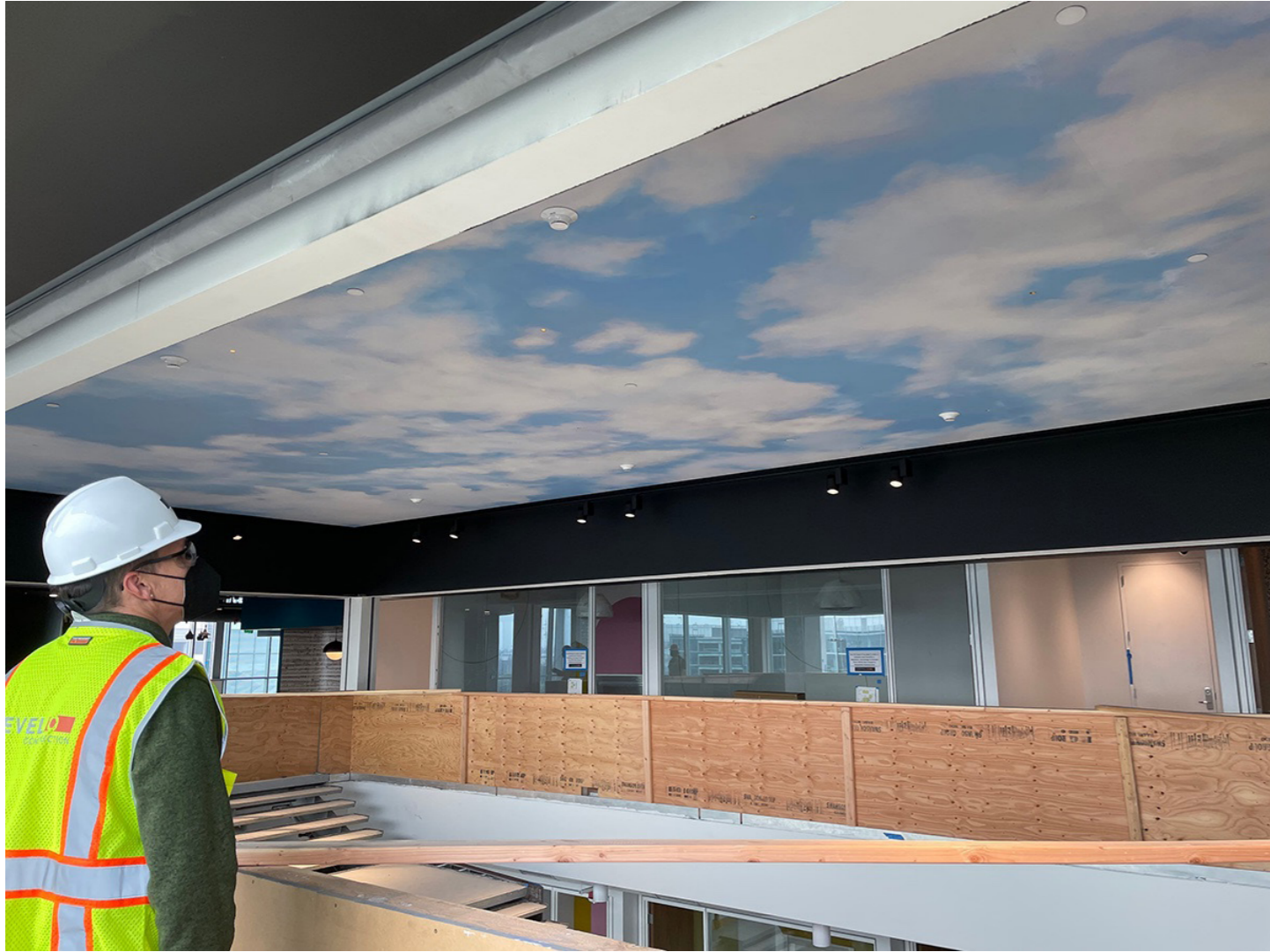
INSTALLATION OF "CLOUD CEILING."
